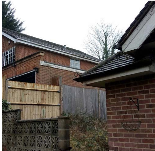
(Photo A – Site Photo of Flank Elevation of 61A)
